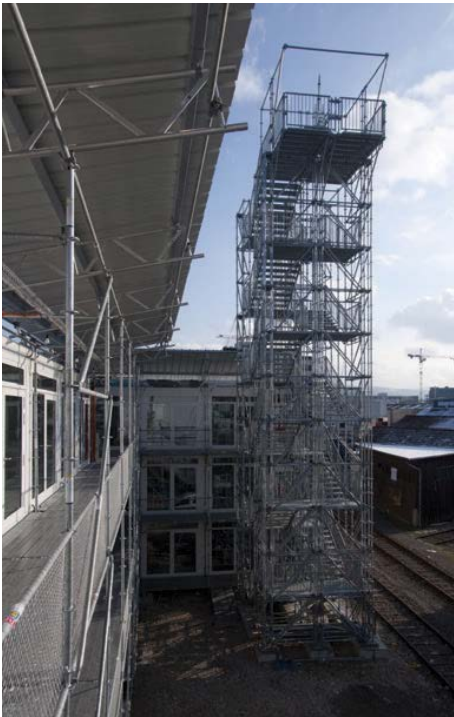
The Rakete (Rocket) project in an industrial area of Basel Switzerland provides temporary space for creative artists and start-up entrepreneurs using shipping containers and scaffolding style stairs and walkways. Photos courtesy of: Christoph Merian Stiftung, Basel
