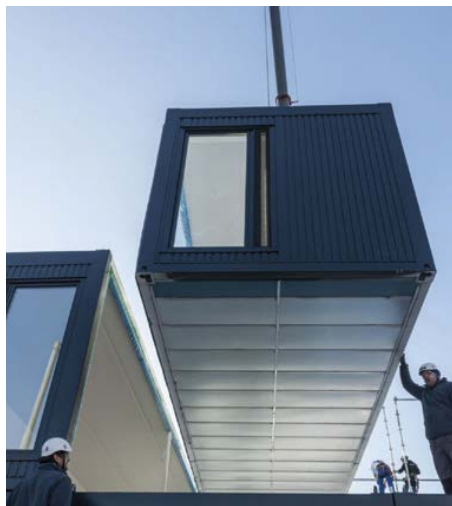
One technique for creating temporary pop-up architecture is to use modular components such as trailers or shipping containers. Photo courtesy of: Christoph Merian Stiftung, Basel
